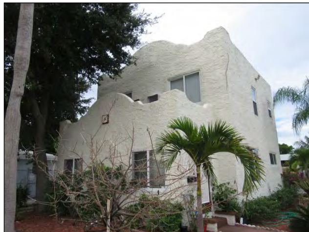
Figure 18. Example of the Mission style. Resource 8PB00493, facing southwest.
