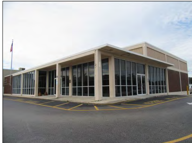
Figure 21. Example of the Modernist style. Resource 8PB16400, facing southwest.
