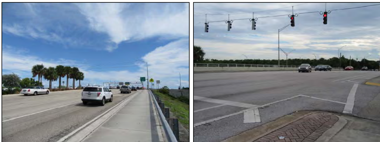
Figure 3. Overview of the development within the Boynton Beach Boulevard and Gateway Boulevard Interchanges APE. Gateway Boulevard over SR 9/I-95, east view (left); Boynton Beach Boulevard over SR 9/I-95, northeast view (right).
