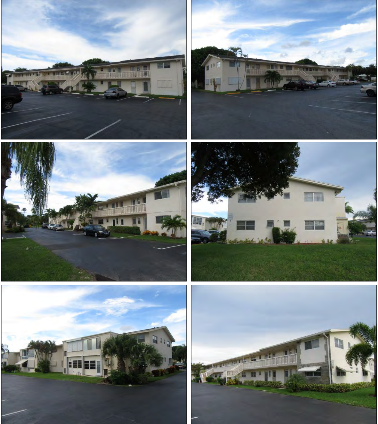
Figure 25. Resource 8PB16399: Building 22 facing northeast (top left); Building 21 facing northwest (top right); Building 19 facing northeast (middle left); Building 17 facing east (middle right); Building 18 facing northwest (bottom left); Building 18 facing southwest (bottom right).
